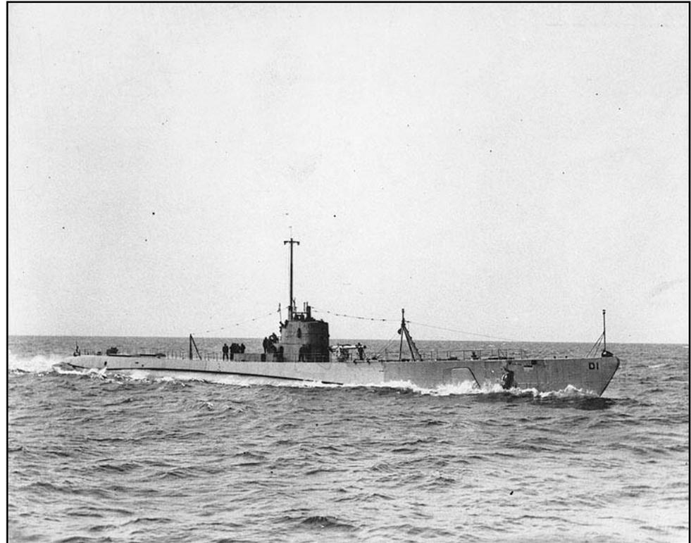
❖ Armament: 6 × 21" torpedo tubes (four forward, two aft), 18 torpedoes, 1 × 4"/50 cal deck gun.
